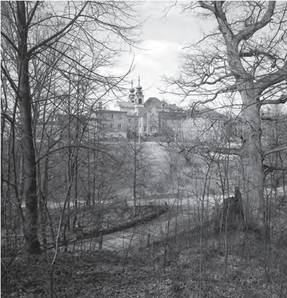
Fig. 2. The Academy of the Catholic Theology buildings in 1970s (Phot. Archive of the UCSW in Warsaw).
